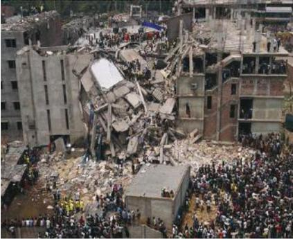
Fig.1. Collapse of 8 storey monolith building in Savar (Dhaka District, Dhaka, Bangladesh)
