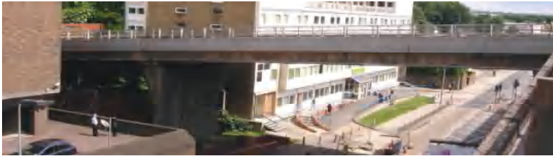
Figure 1. General view of the Pentagon Road Bridge
