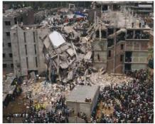
Fig.1. Collapse of 8 storey monolith building in Savar (Dhaka District, Dhaka, Bangladesh)
